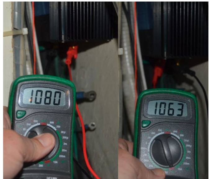
Figure 7. Testing a Galvanic Isolator
